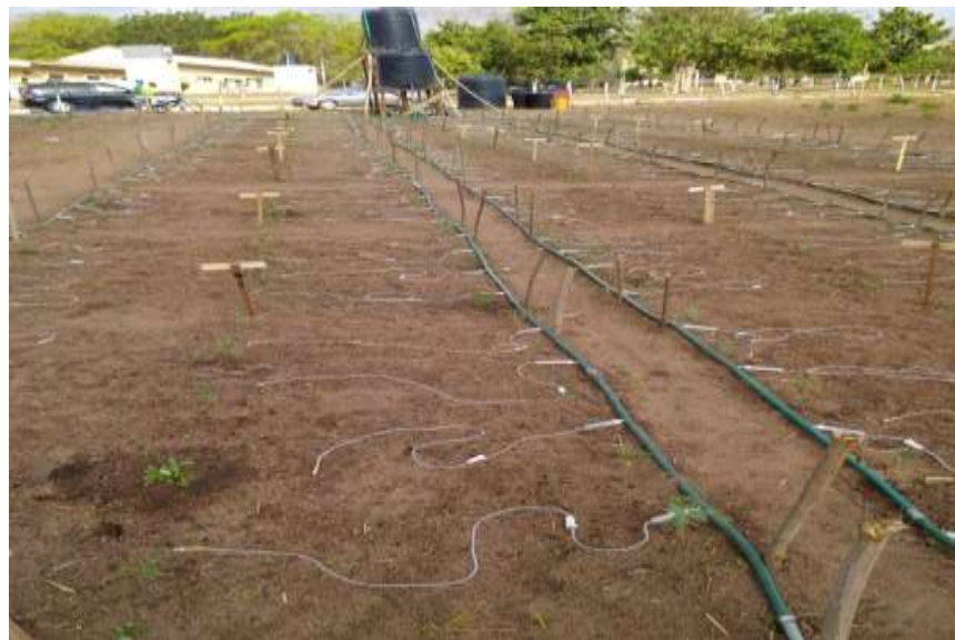
Plate.1: The drip irrigation setup showing the medi-emitters
